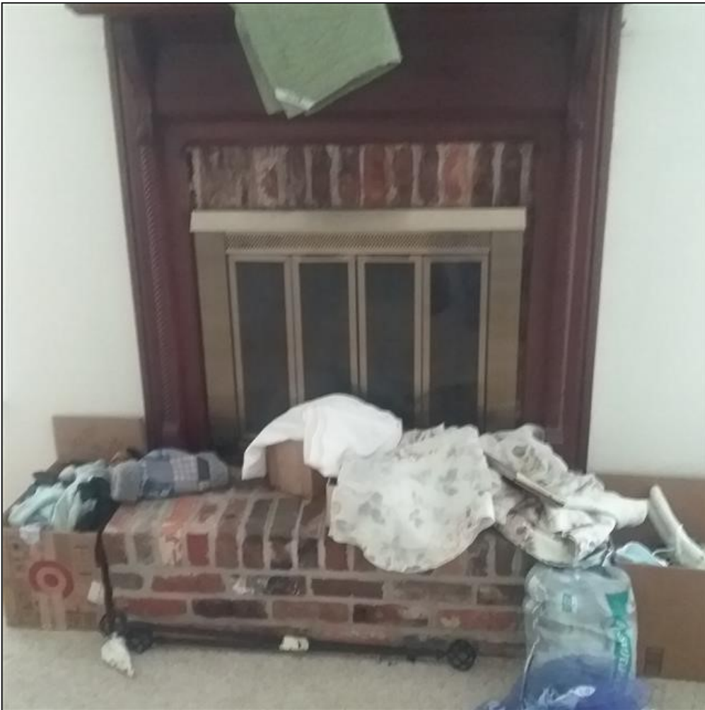
8.7 Item 2(Picture) Front right bedroom is a conventional fireplace.
