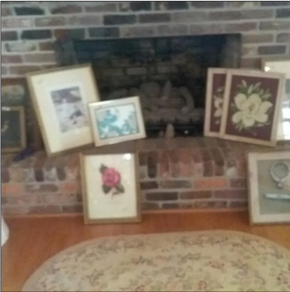
8.7 Item 1(Picture) Vent less gas logs main room.
